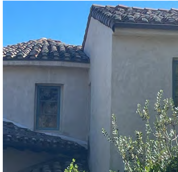
Figure 50: Example of a complex roof, which introduces several locations where flammable debris and embers can gather.
