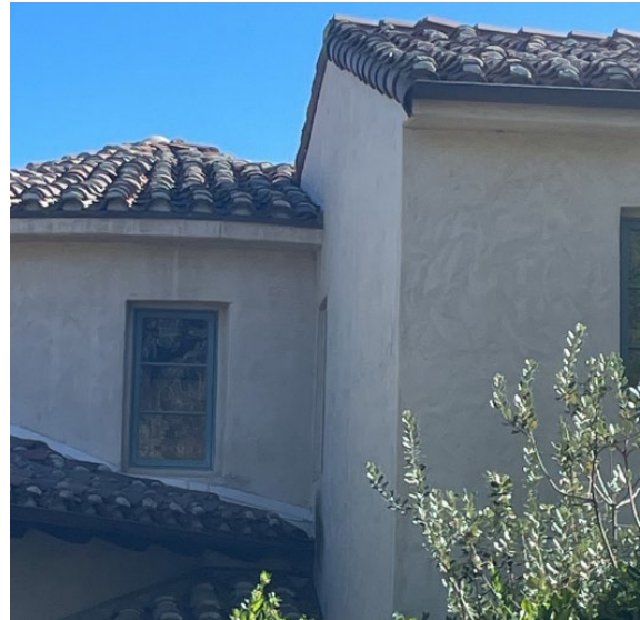
Figure 58: Example of a complex roof, which introduces several locations where flammable debris and embers can gather.
