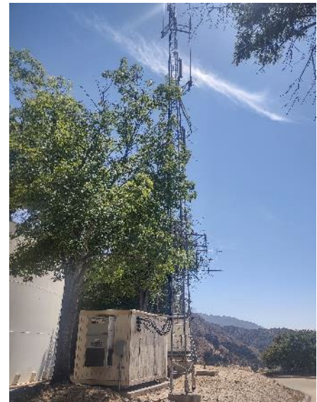
Figure 66. Water and communications infrastructure in a wildfire prone area.
