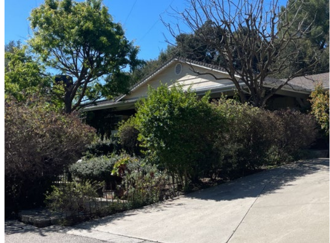
Figure 56: Overgrown vegetation in Zone 0 and 1 proximate to the exterior of the home. This introduces several paths for fire to spread and encroach the home.
