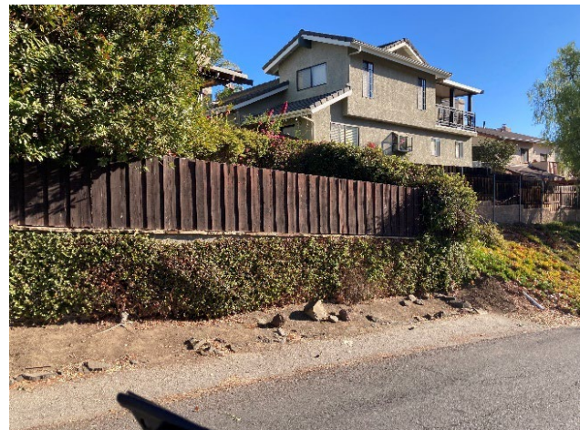
Figure 57: Wooden fences and vegetation near and between homes can act as a “wick” that contributes to fire spread.
